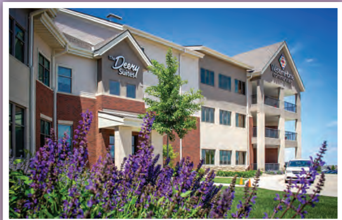
The new SFAL at Deery Suites is located on the first floor and includes the patio seen at far right.
